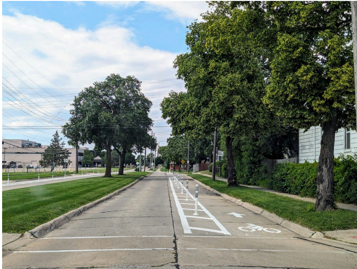
Separated Bike Lanes on boulevard section of Lawrence Street in Center Line
