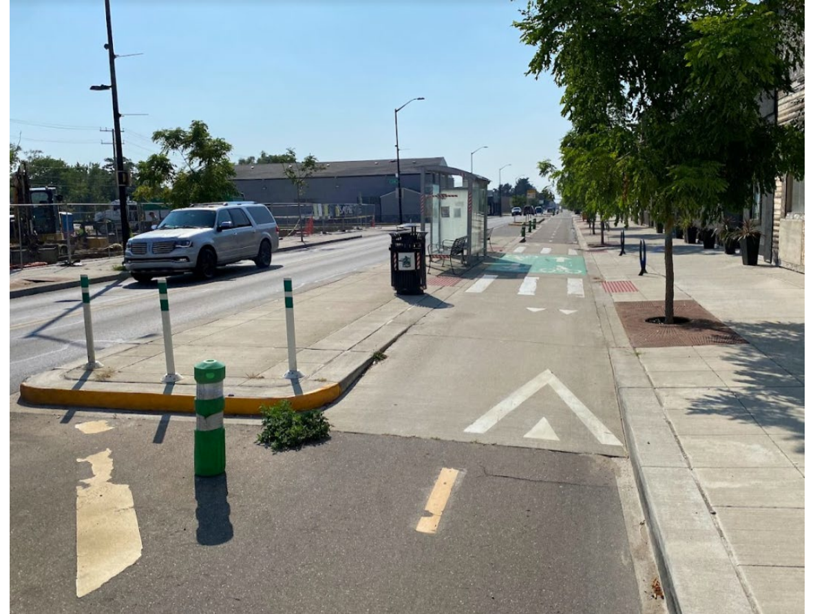
Two-Way Separated Bike Lane on McNichols in Detroit
