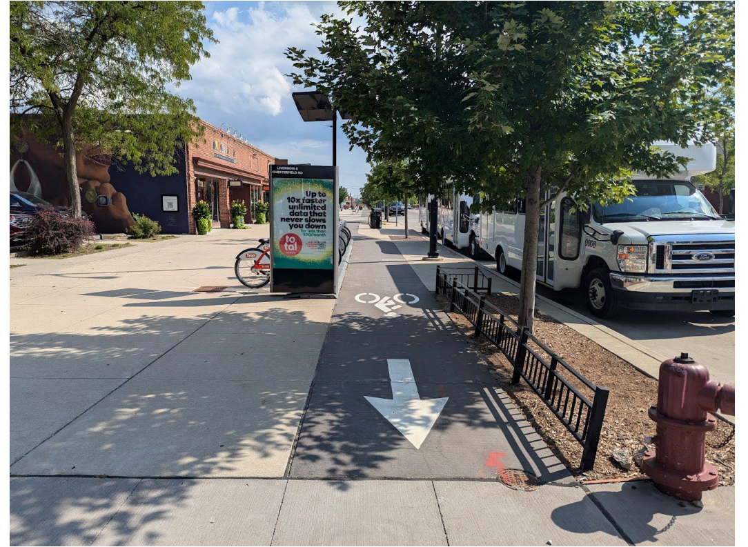
Raised and Separated Bike Lane on Livernois in Detroit
