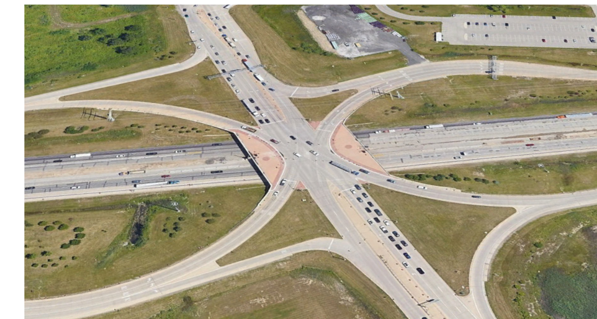
Establish high quality non-motorized link through the Beck Road overpass
