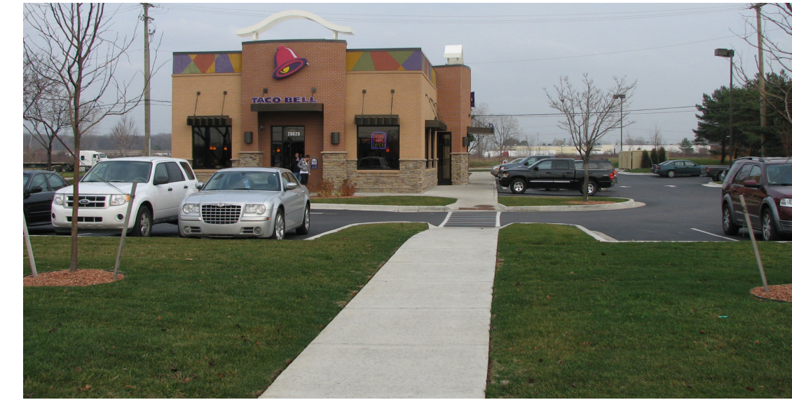
Provide access from the public pathways and bike lanes along the street to the business' front door
